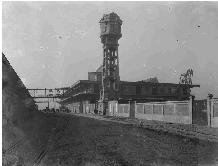
Katoenveem, view from Keilestraat around 1920. Visible are the water tower, railroads, cranes, transportation bridges to warehouses 'New Orleans' and 'Galveston' and the walled outside storage space. Photo from Historisch Centrum Overijssel (retrieved 24-10-2016).
