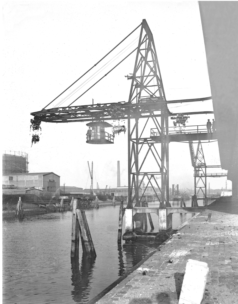
The cranes were connected to the transit system inside the Katoenveem, Historisch Centrum Overijssel (retrieved 24-10-2016)
