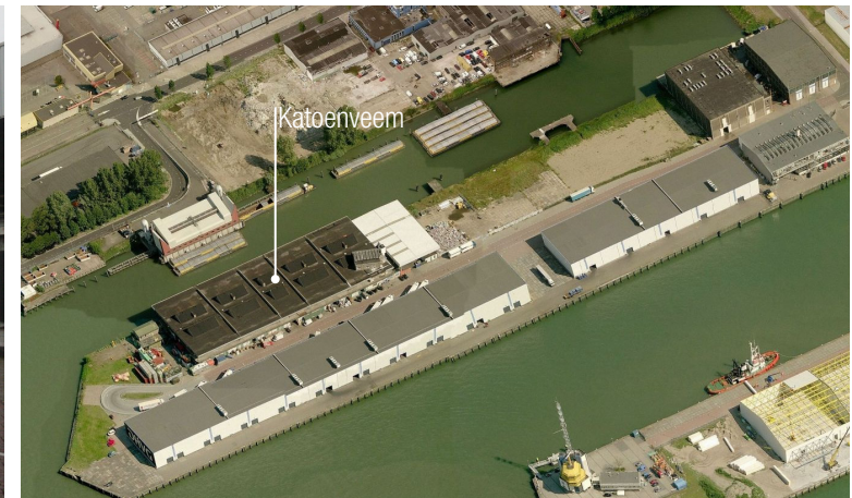
Aerial view of the current situation of the Katoenveem and its surroundings. Bing maps (retrieved 24-10-2016).
