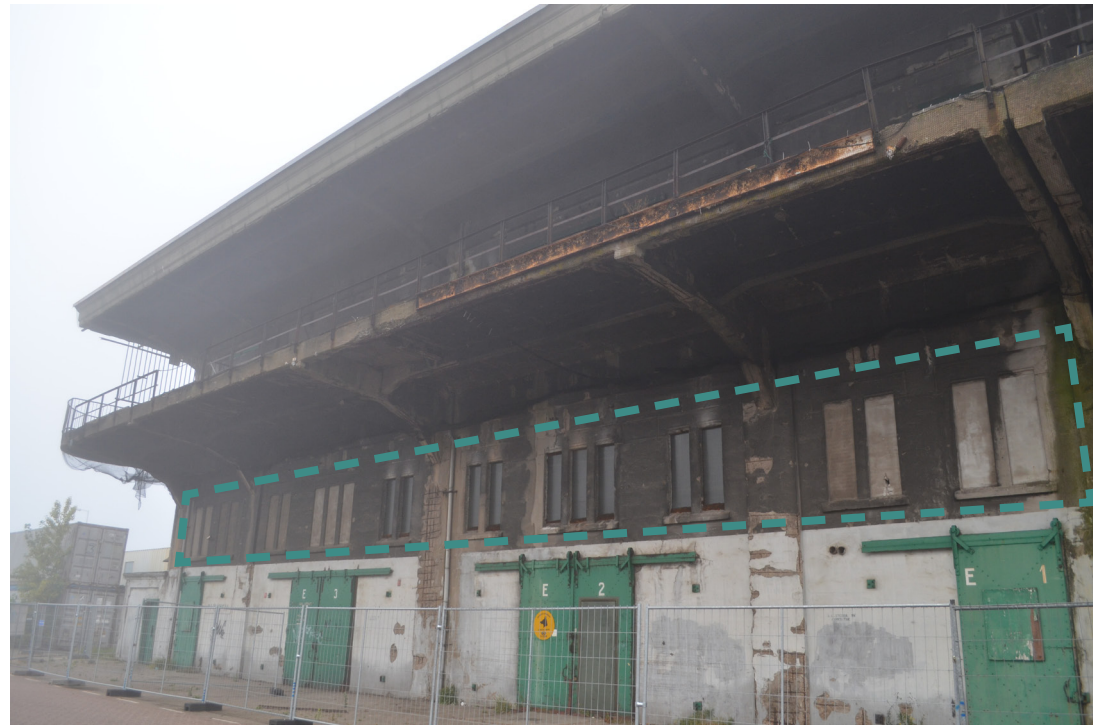
Windows under the balcony. Many of them are closed, own photo (2016).
