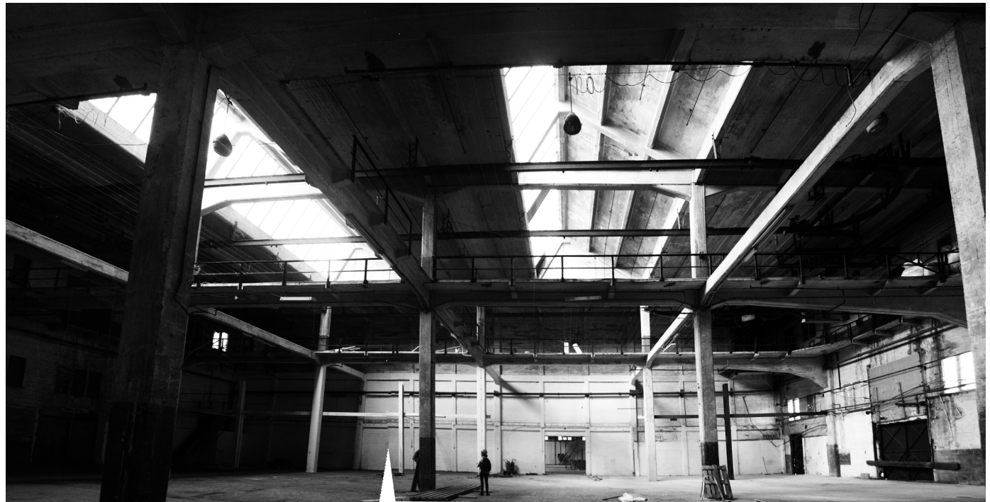
A great portion of the daylight entered the building through the roof lights, creating a pleasant space for working, own image (2016).
