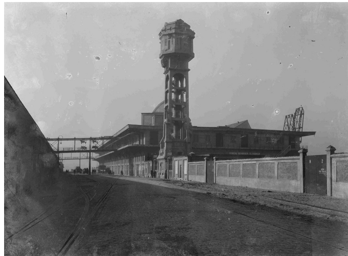
Image 2: Katoenveem in 1921, just after completion. Visible are the water tower, transporting bridges, cranes on the waterfront and outside wall. Source: Historisch Centrum Overijssel
