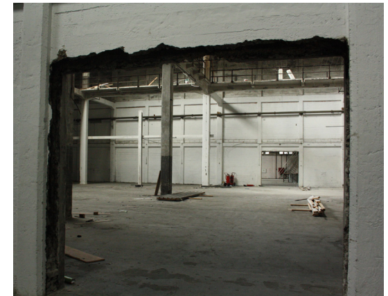
Interventions: addition of a steel structure, closing of the windows and creation of passageways through the fire walls. Photos by students (20-09-2016).
