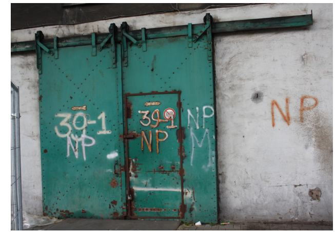
Large steel sliding doors on the ground floor, own photo (2016)
