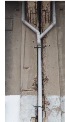
Rain pipes, own photo
