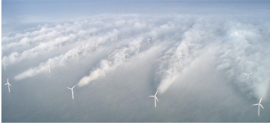
**Figure 1-3:** Horns Rev 3 is an offshore wind farm situated near Denmark. Turbulence introduced as a result of aerodynamic interactions between the wind turbines can be clearly seen. Source: Vattenfall [3]
