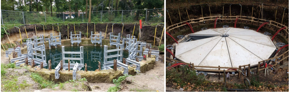
Figure 8.3: Construction of the STESS. Left: installation of the last heat buffer. Right: STESS almost completely sealed.
