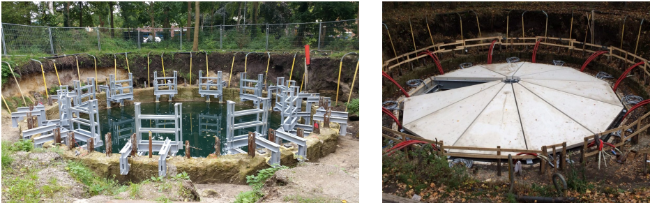
Figure 7.2: Construction of the real Ecovot system.
