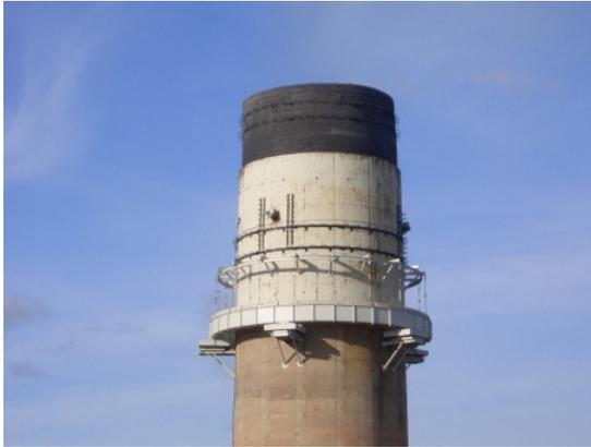
**Figure 2.15:** Tuned mass damper of 41 tonnes installed on top of a 180m concrete chimney [2]
