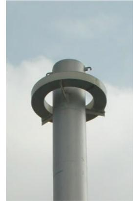
**Figure 2.16:** Liquid damper on top of a 100 m steel stack used also as a top platform [2]
