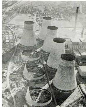
**Figure 1.1:** Three collapsed towers in Ferrybridge, UK [49]
