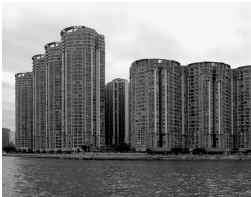
1 Concentrated high-rise development in Hong Kong, China.
