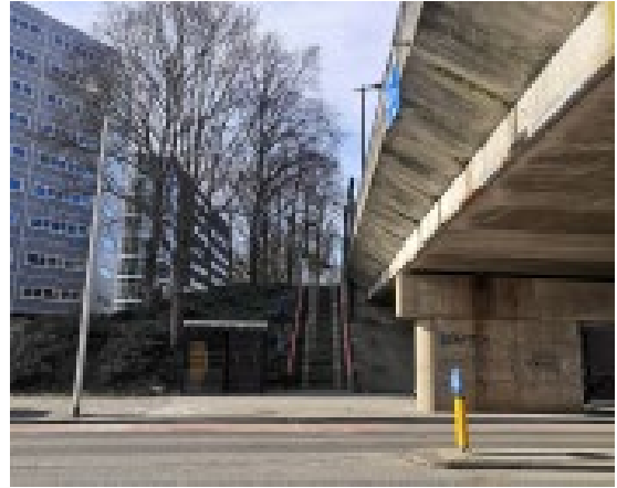
Dikes for infrastructure and buildings pose barriers in pedestrian flows
