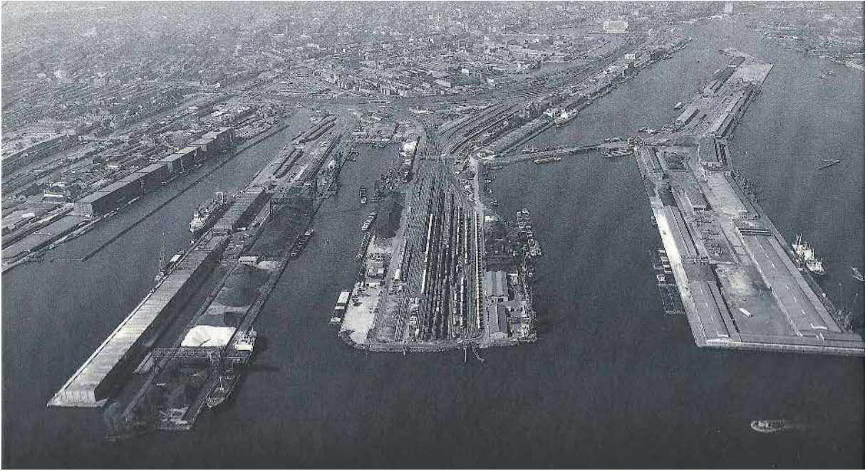
FIGURE 2 Eastern Harbor Area Amsterdam: 1960s. Source: West 8 (60s)
