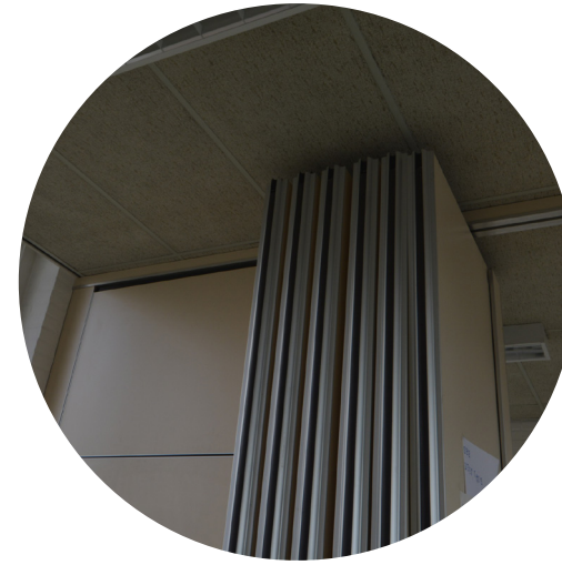
interior walls | movable wall panels
