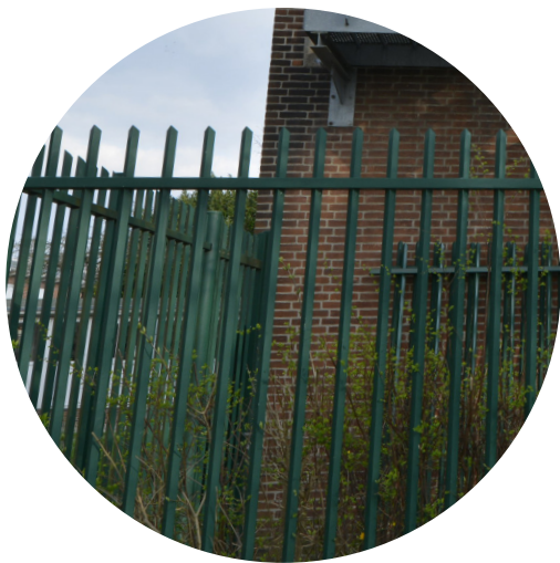
plot fencing | steel painted green
