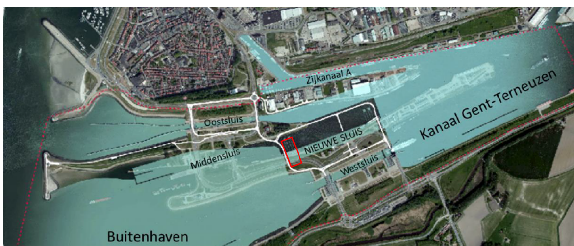
Figure 1.1.1: Top view of the project area that represents the previous and current situation of the Locks in the Gent-Terneuzen canal (SSV-RAP-163-C project report).
