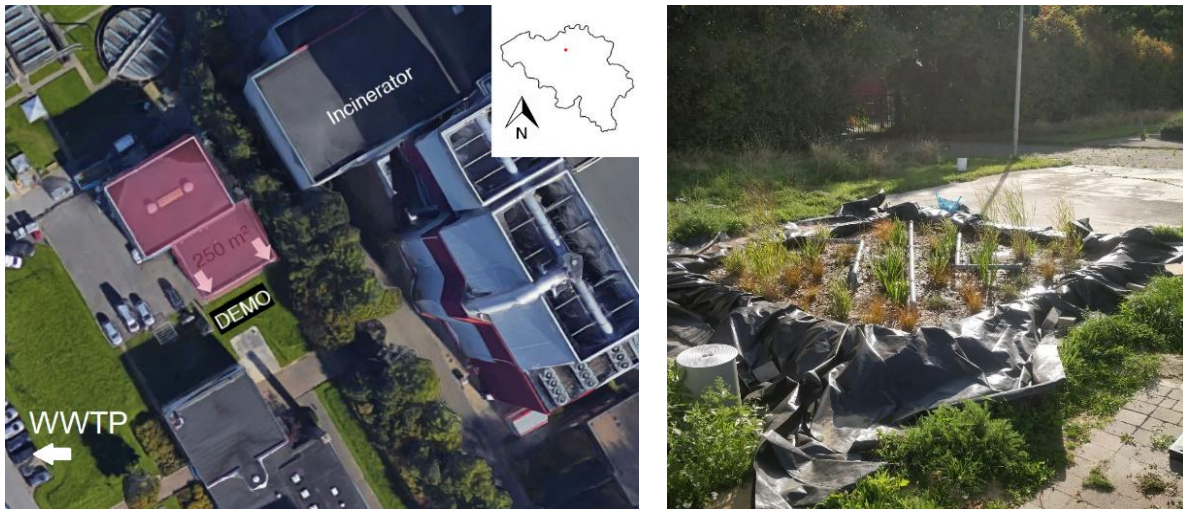
Figure 3-1 Location of the Aartselaar demo (51°08'51.1"N 4°22'32.1E). Roof water catchment highlighted in red (left). During the field experiments, the demo was operated without concrete edges up to November 2019 (right) (Versteeg, 2019).
