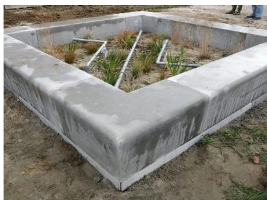
Figure 3-3 Left: Final design of the BB with concrete edges. Water was distributed onto the BB by three sprinkler pipes (Versteeg, 2019) Right: During operation the water level rises and mimics a wetland. Demo Aartselaar 19 th of September 2019 (Versteeg, 2019)
