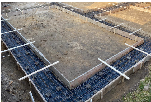
Figure 5.1: Cast-in-situ shallow strip foundation process [31]
