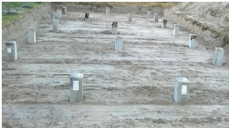
Figure 3.17: Regular prefab prestressed house pile plan
