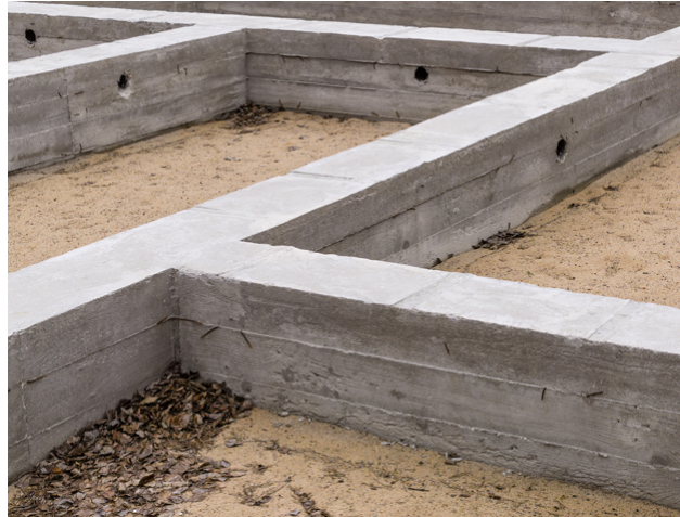
Figure 3.18: Shallow strip foundation variant [28]
