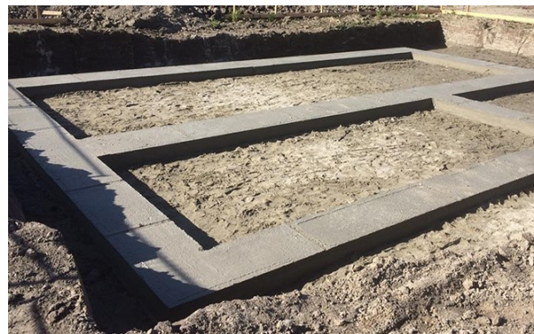
Figure 5.2: Shallow concrete strip foundation [31]
