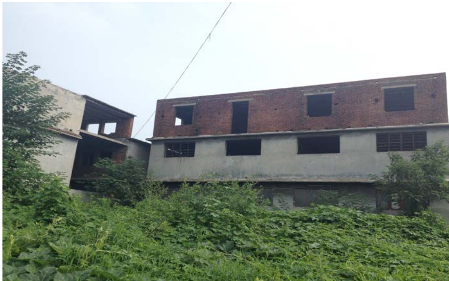
Figure 22 Additional floor on top of the original house in Nanzhang village, Yanzhou, Shandong
