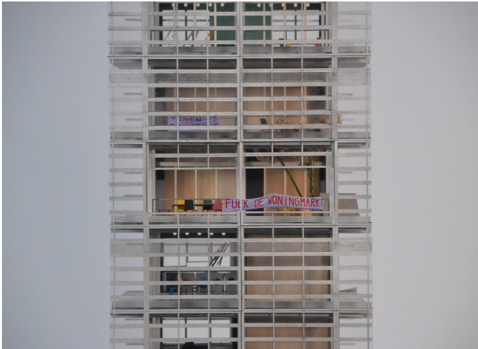
south facade detail
