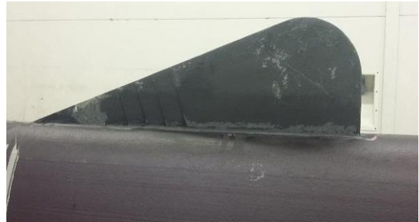
Assembly of Lug Plate on Mast
