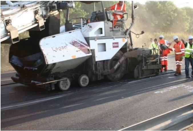
Figure 4. Paving process of the trial section (2)
