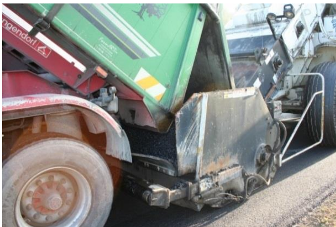
Figure 3. Paving process of the trial section (1)
