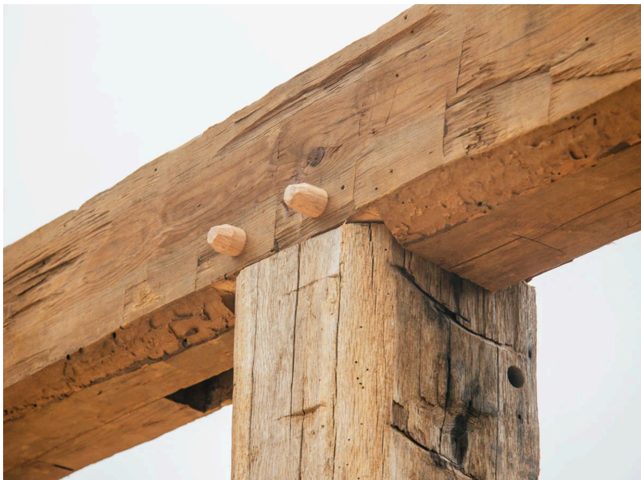
Figure 3.8: A Pegged Mortise and Tenon joint connecting a Beam to a Post
