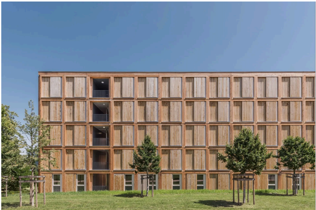
Figure 1.4: The Rigot Collective Dwelling Centre in Geneva was built to quickly house 370 refugees. Constructed from prefabricated wooden modules, this two-building complex is designed to be taken down within ten years.
