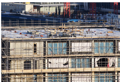
Start of the extension with the steel bases (Skyscrapercity, 2012)
