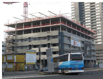
Steel frame top up in construction (Skyscrapercity, 2012)
