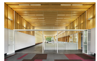
North Vancouver City Hall, featuring mass timber LSL panels, by MGA Architects in Vancouver, Canada. (StructureCraft, 2014)
