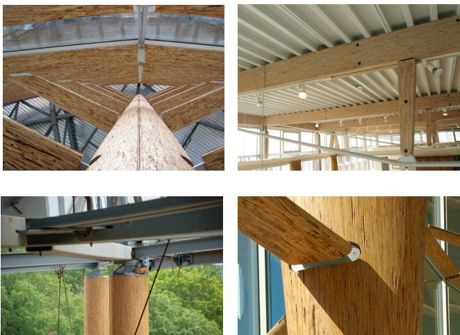
PSL can be manufactured in many shapes and used in different applications. These are some examples in combination with steel intermediary connections or steel composite beams (StructureCraft)
