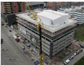
Topping out of the structure with the facade going up (Skyscrapercity, 2012)
