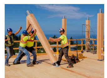
The structure could be erected by hand due to the light weight nature of timber (Fast, 2016).
