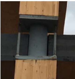
Picture of the column floor connection (Poirier, Moudgil, Fallahi, Staub-French, & Tannert, 2016)
