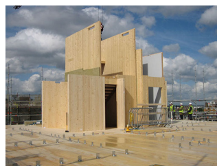
Photo illustrating the bracket connections and the stairwell (KLH)
