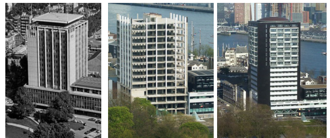
On the left the old Vopak building, in the middle the stripped building, on the right the finished renovated Westerlaantoren
