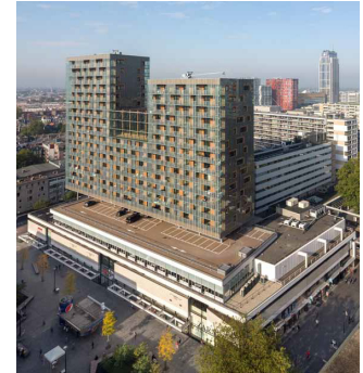
The finished building on top of the old Ter Meulen building (Ibelings & van Tilburg, 2013).
