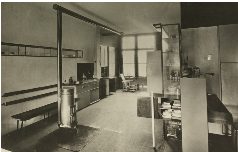
Figure 26. The flat of An and Rein Harrestein in Amsterdam. Truus and Rietveld created the design together (Rietveld Schröderarchief, n.d.).
