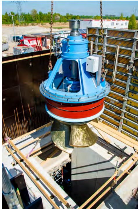
Figure 4.30: Hoisting of a CVP Impeller Blade and Bearing (Van Der Ven, 2020)
