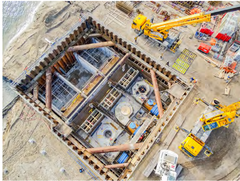
Figure 4.4: Preparation of the Casing for a CVP (Van Der Ven, 2020)
