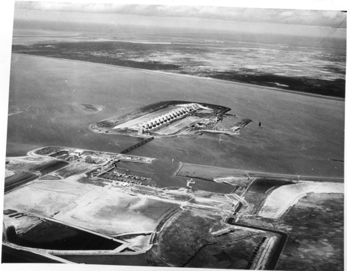
Figure 7.1: Construction Pit for the Haringvlietdam (Slagboom, 1965)
