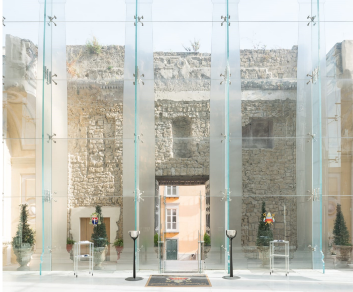
Figure 19a. The ruins of the Augustan Temple in Pozzuoli (Italy) are restored with a glass façade that consists of fins and plates outlining the shape of the original columns (Gnosis Architettura and Bardeschi 2017)
