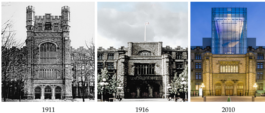
Figure 18. The original tower of the Victoria Memorial Museum in Ottawa had to be removed due to unstable soil conditions and its massive weight and was replaced by a glass tower after the rehabilitation of the monument into the Canadian Museum of Nature in 2010 ( https://nature.ca/en/about-us/history-buildings ).
