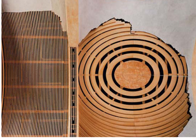
Figure 2c. The new roof of San Filippo Neri in Bologna (Italy) uses wood, a traditional material, in a rather contemporary way to preserve the outline of the collapsed part due to Second World War bombings (wegstudio 2018).
