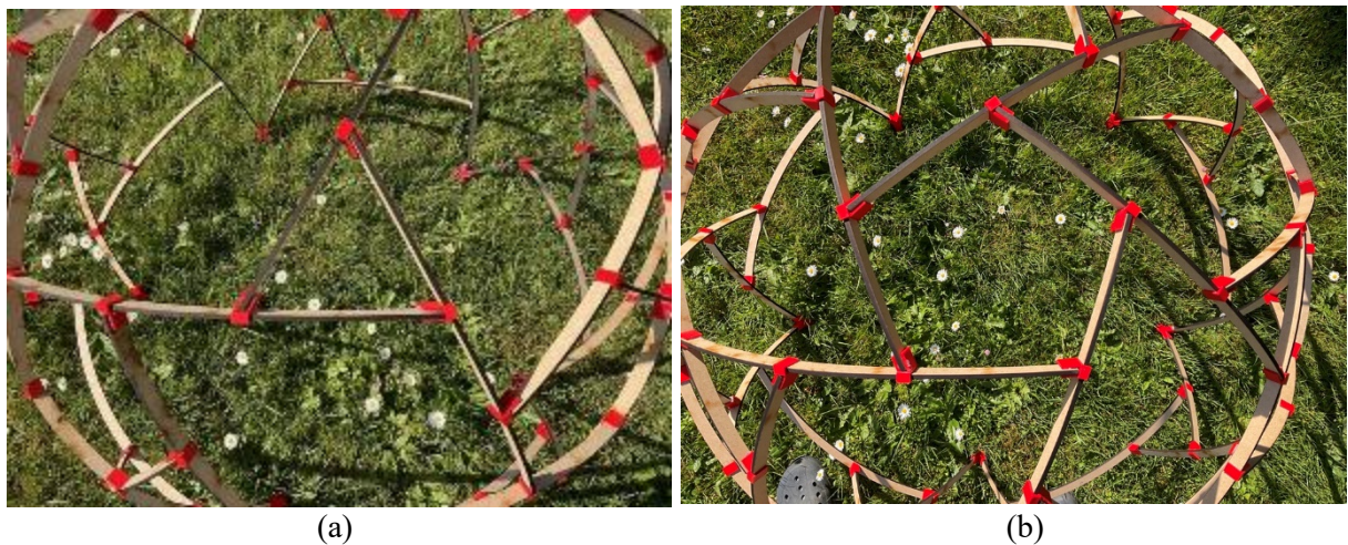
Figure 11. (a) Triangles and (b) pentagons formed by respectively the Type 60° and Type 108° connectors.
