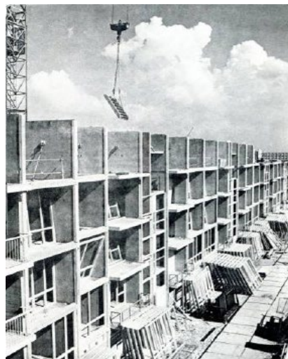
Figure 7. Construction of Intervam flats (Priemus & Van Elk, 1971)
