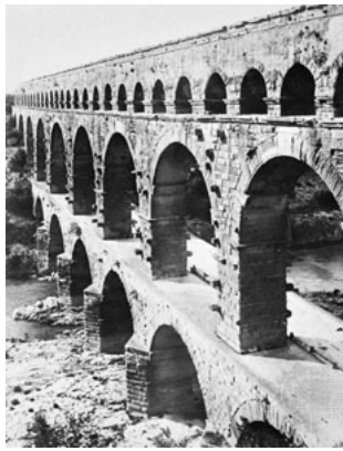
(a) Pont du Gard - vault arch structure (Nîmes - France)
