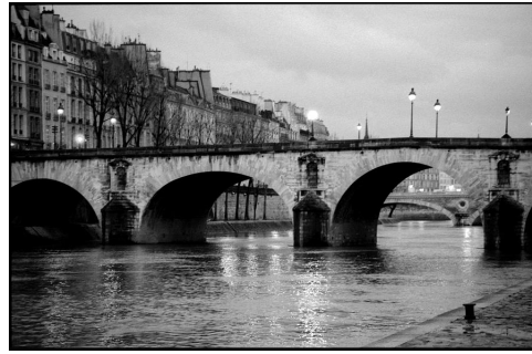
(b) Pont Royal - elliptical arch structure (Paris - France)
