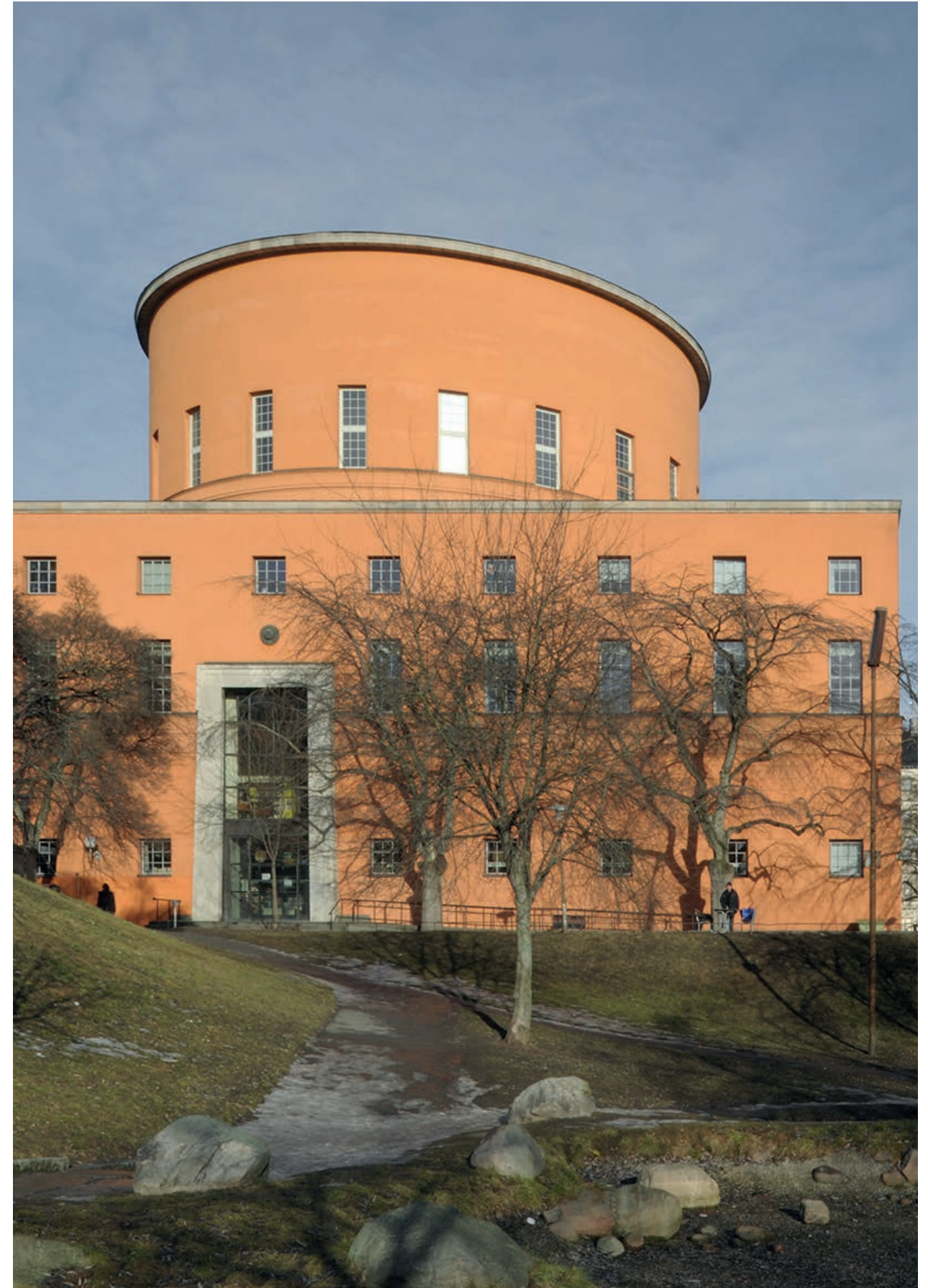
Archival photo view towards the south entrance, Stadsbibliotek Stockholm, by David Grandorge 01
