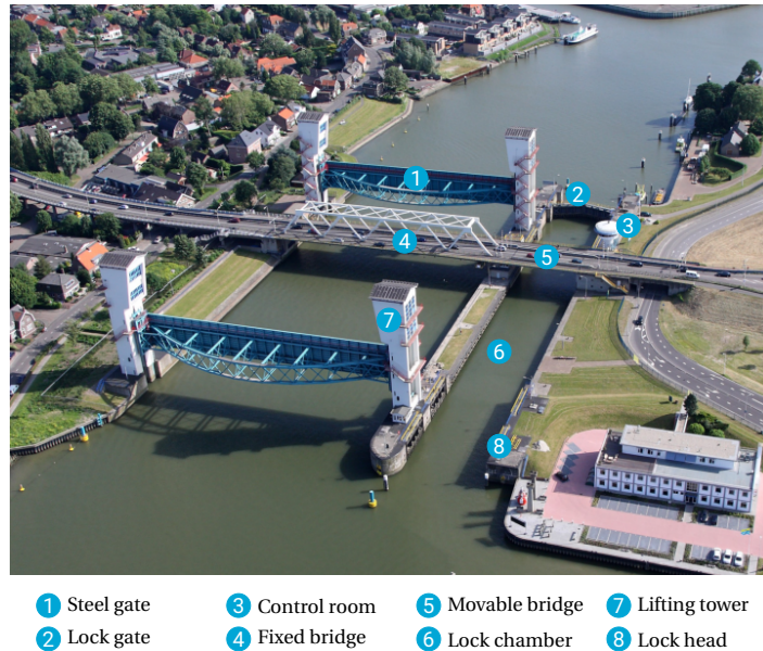
Figure 2.11: Overview of several elements of the Hollandsche IJssel barrier, picture by Van Houdt (2008).
