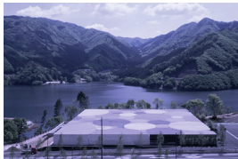
TOMIHIRO ART MUSEUM Location: Midori, Japan Architect: aat + makoto yokomizo GFA: 2 463 m 2
