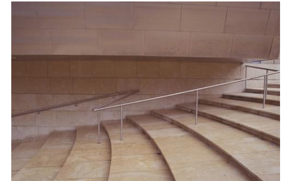
Fig. 28: Guggenheim, Bilbao Entrance area - iconic architecture creating disfunctional spaces
