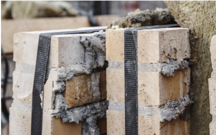
storing cut out brick panels © Lendager
