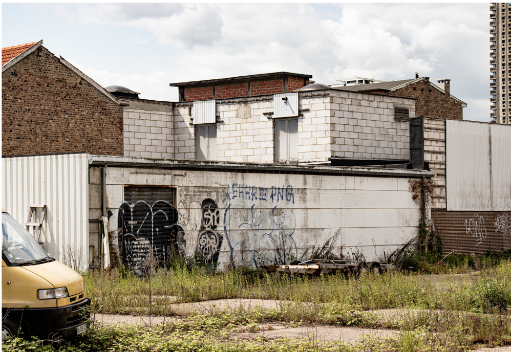
concrete masonry, brick masonry, corrugated sheeting, roller door, roof light, timber framing (picture by author)
