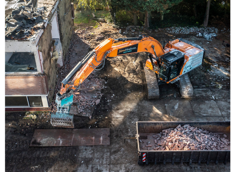
seperating bricks during demolishment © New Horizon
