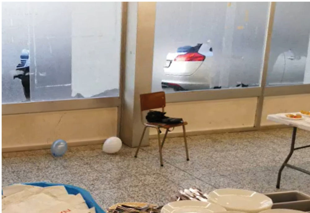
curtain wall, floor tiles (image courtesy of Int. Church of Pentecost)
