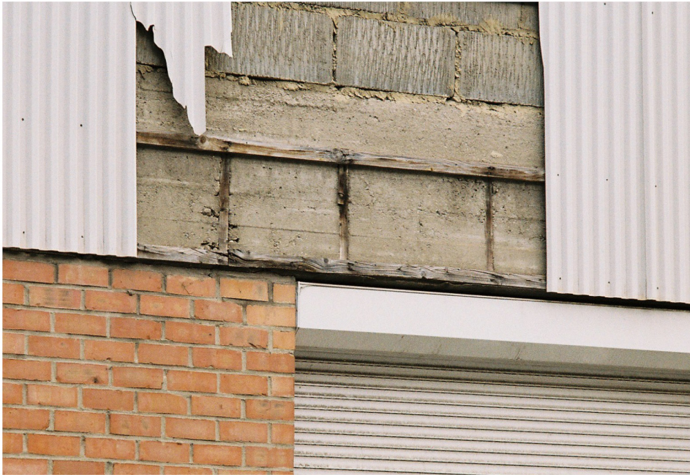
brick masonry, concrete masonry, corrugated sheeting, roller door (picture by author)
