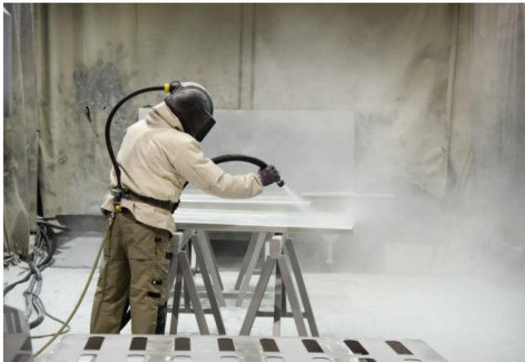
sandblasting steel structures © coating.nl
