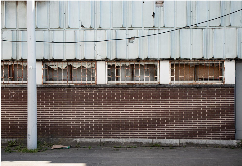
brick masonry, window grill, window frame, facade panel (picture by author)
