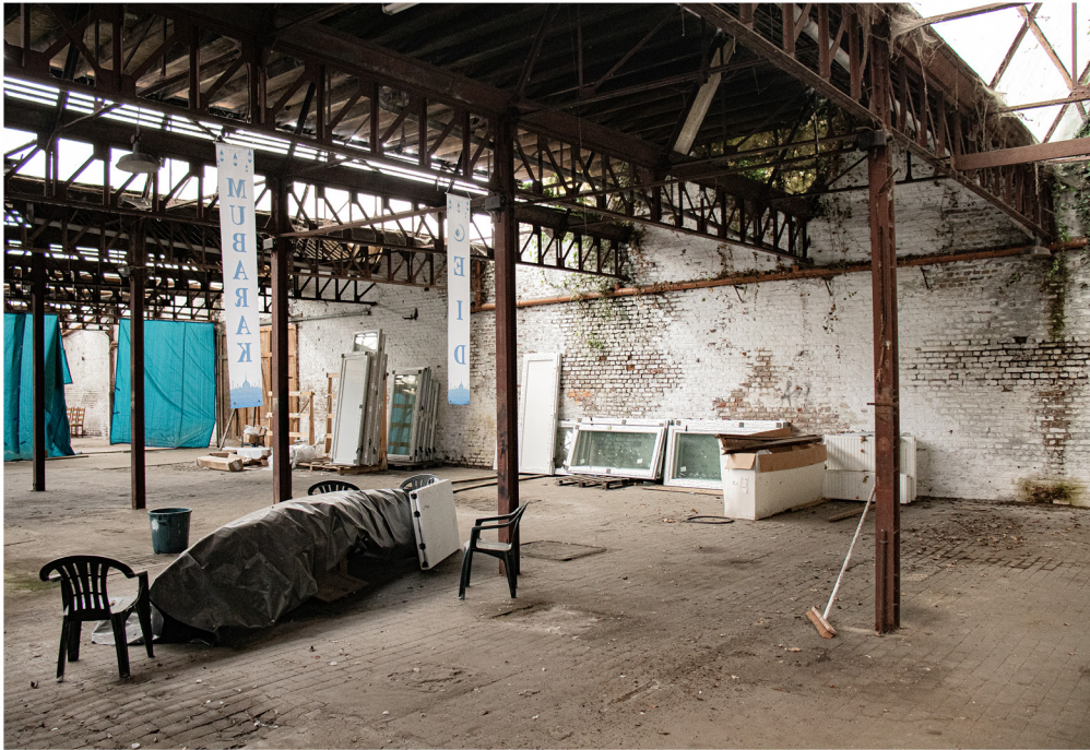
brick masonry, column, straight truss, dual pitch truss, timber framing, paving tiles (picture by author)
