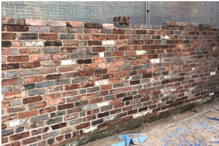
reuse of reclaimed bricks © SalvoWEB
