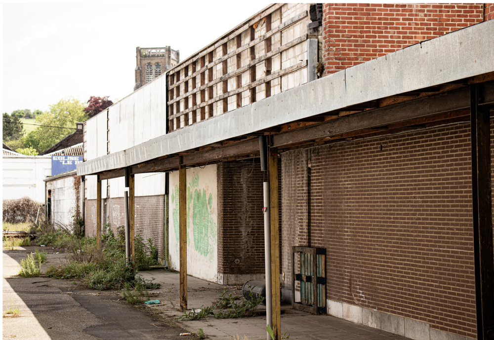
corrugated sheeting, brick work, timber framing (picture by author)
