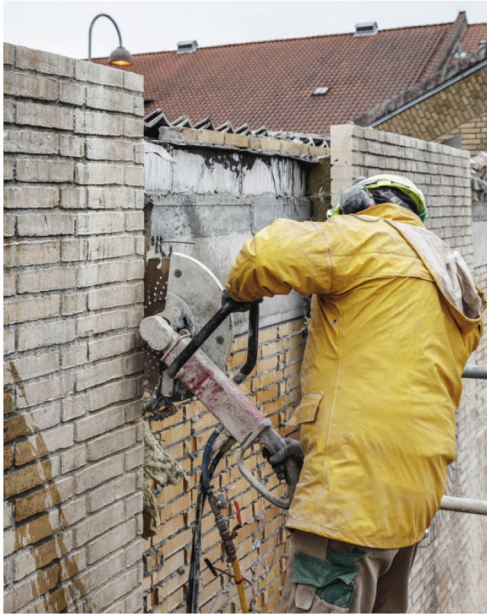
cutting out a brick panel © Lendager
