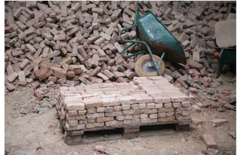
sorting bricks on site © FCRBE
