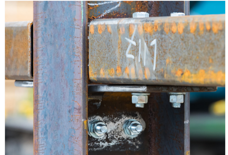
application of reused steel constructions © Circulair Staal
