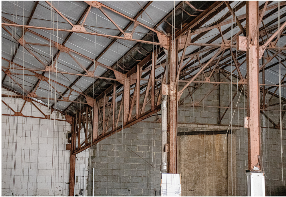
concrete masonry, pitched truss (picture by author)
