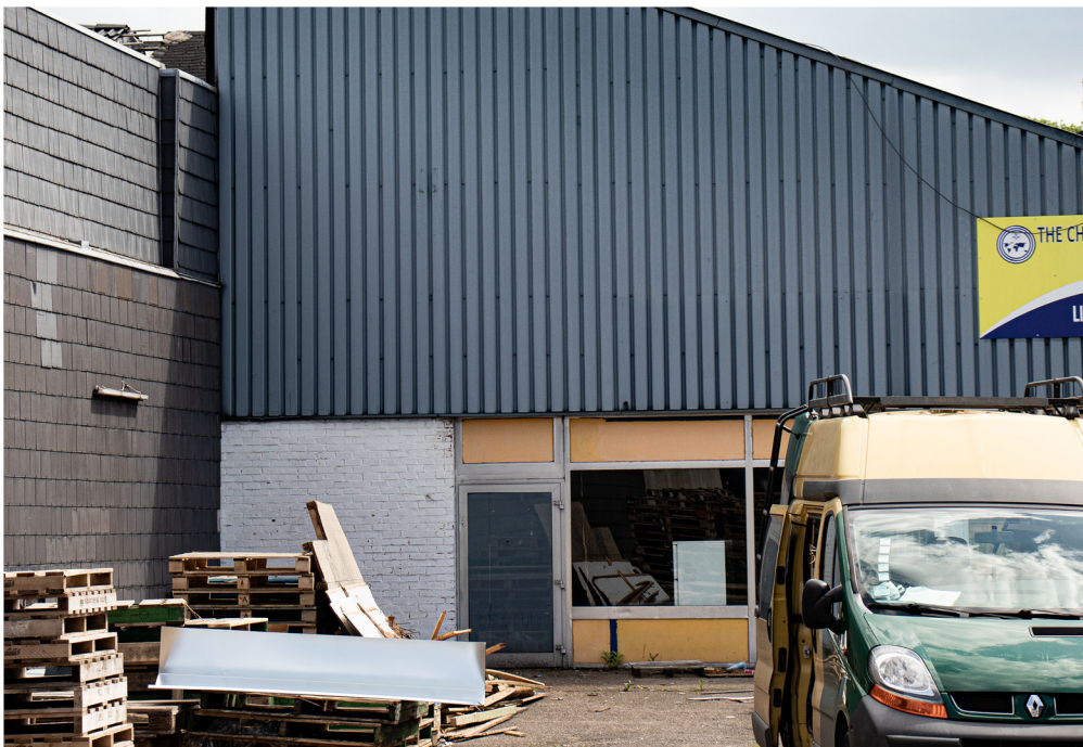
brick masonry, corrugated sheeting, curtain wall (picture by author)
