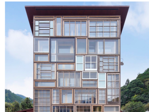
application of remanufactured window frames Kamikatz Public House, © Hiroshi Nakamura & NAP
