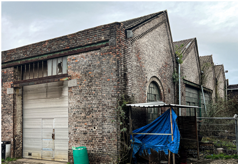
brick masonry, ceramic roof tiles, roller door, window frames (picture by Simon van Sooling)
