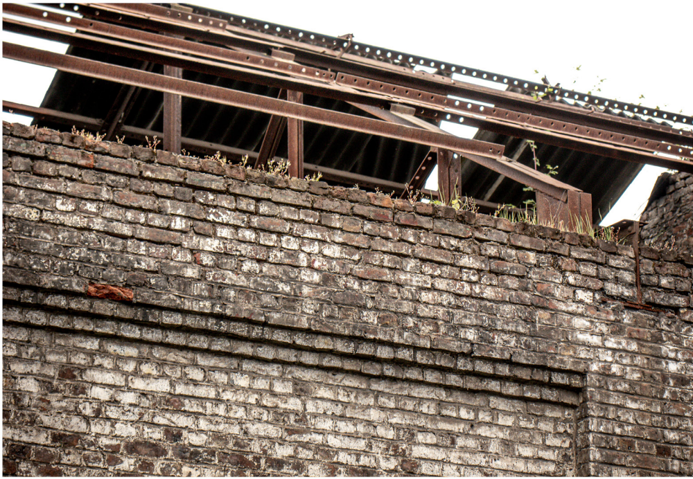
brick masonry, pitched truss, steel frame work (picture by author)
