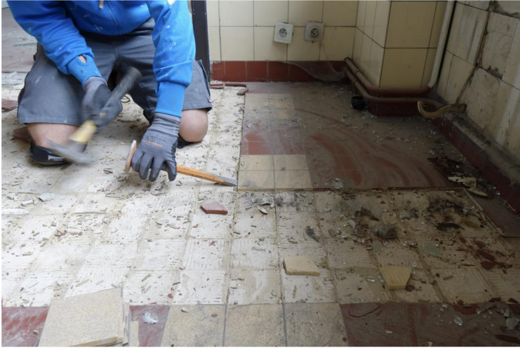
removal of re-useable ceramic tiles © RotorDC
