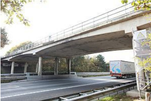
Fig. 1: Photograph of viaduct De Beek
