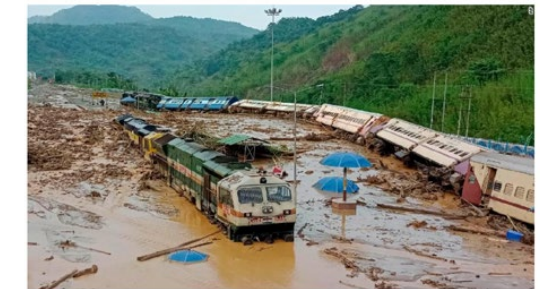
Train coaches toppled over after mudslides triggered by heavy rains at the New Hahong railway station in Assam, India, on May 16.
