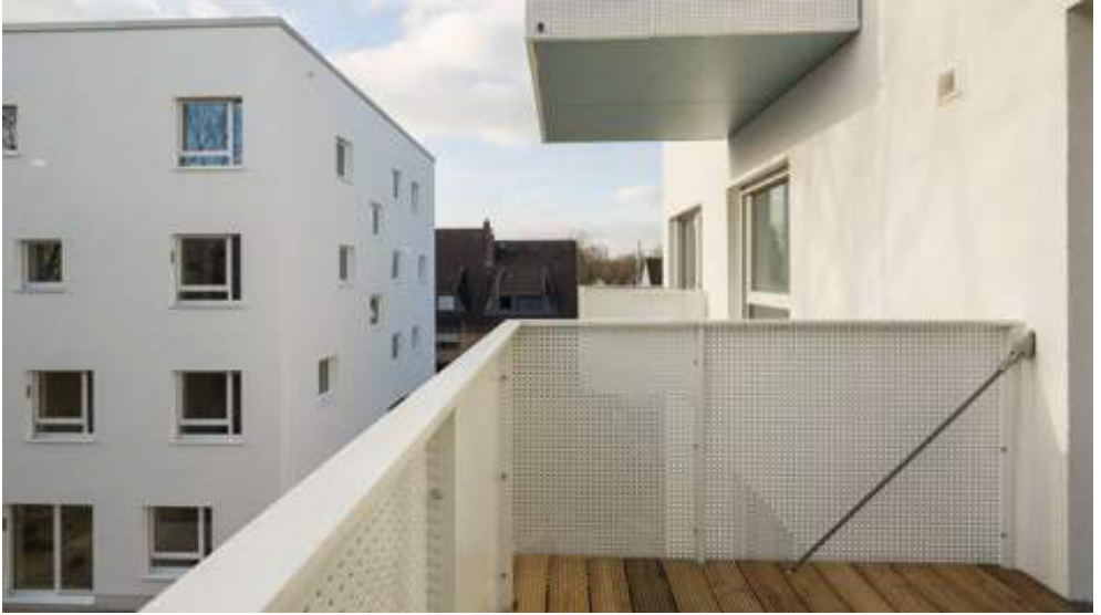
Figure 38: Optional balconies that can be attached and removed whenever the needs arises. (GEWOBA & LIN Architects, 2020)
