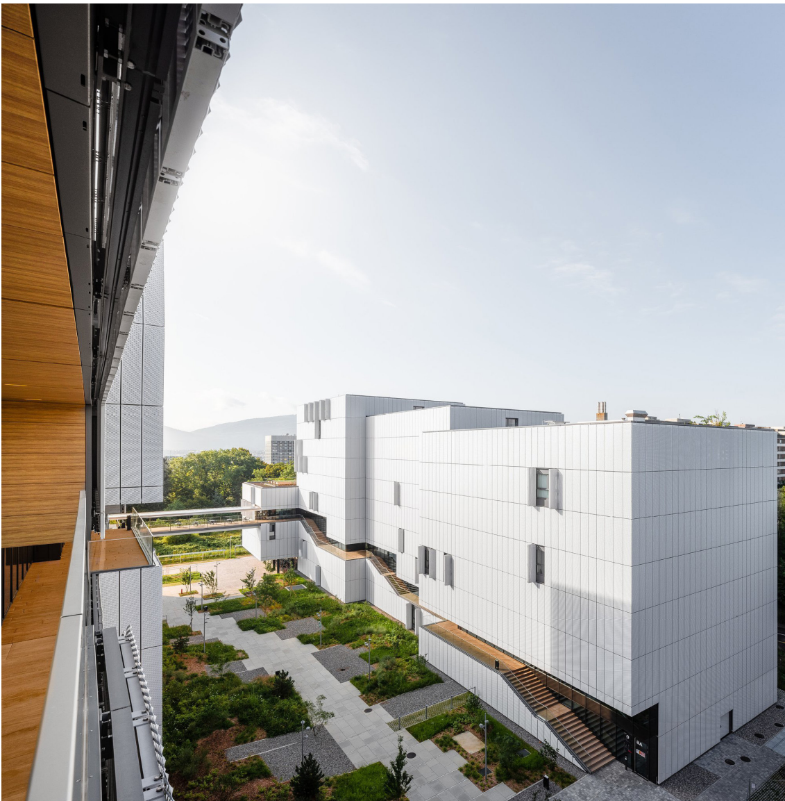
Figure 29: Grand Morillon student residence/ Kengo Kuma & Associates (CCHE, 2021)
