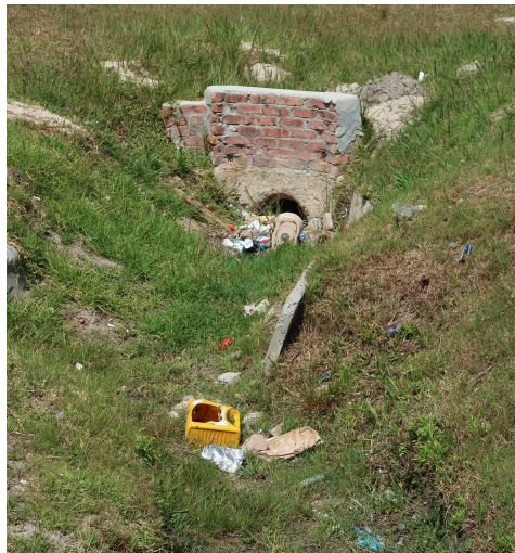
Figure C.6: Outlet structure with debris
