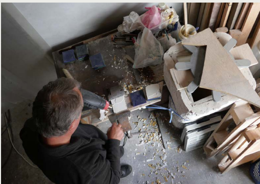
Chipping cement off tiles
