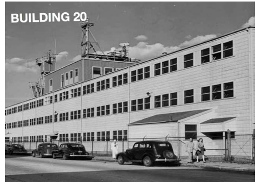
Fig c.4: MIT's Building 20 in Cambridge, Massachusetts. A simple wooden frame made up the main construction.
