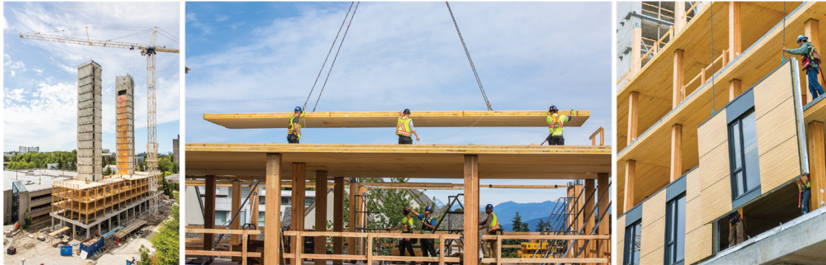
Brock Commons Tallwood House, Vancouver Acton Ostry Architects
