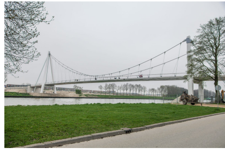
(b) Dutch bicycle bridge - Daphne Schippersbrug
