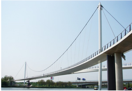
(a) Dutch bicycle bridge - Nesciobrug
