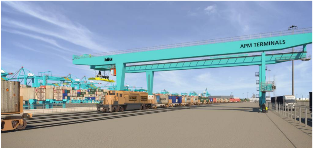
Figure 7.53: APMT Maasvlakte 2 rail terminal with gantry crane, artist impression (source: APMT)
