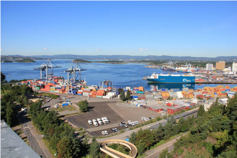
Figure 7.39: Overview of the Ormsund container terminal in the Port of Oslo (source: Port of Oslo)
