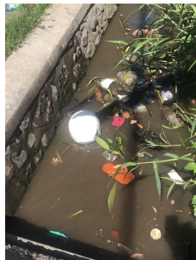
Figure 4.3: Example of Open Drain for Rainwater in Desa Saba
