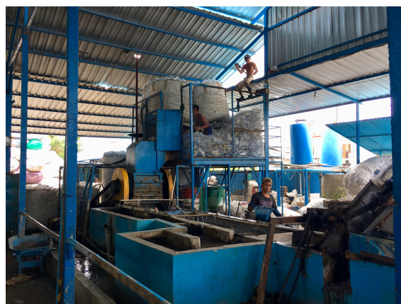
Figure C.4: Production Line in the Bali PET Facility
