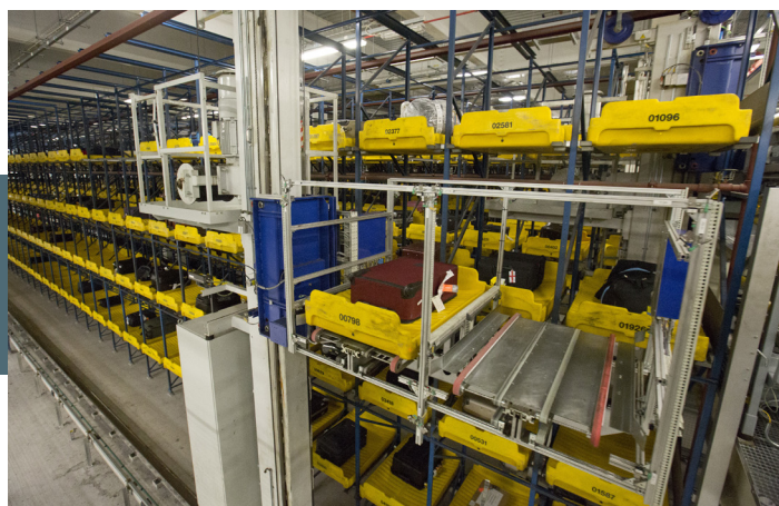
Figure 32: Individual storage in cranes (Source: Vanderlande)
