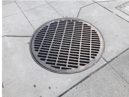
(b) a manhole
