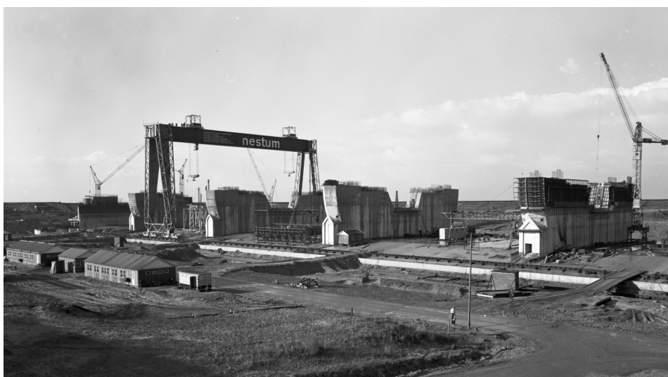
Figure 6.13: Nestum bridge-crane during the construction of the Haringvlietsluices
