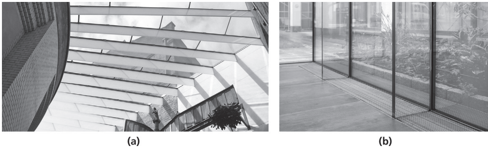
Figure 6.11 Glass plates in (a) glass floor in the New Acropolis Museum, Athens, Greece, and (b) unitised curtain wall facade. (Author's own)
