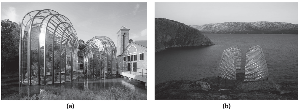
Figure 6.12 Glass shell structure in (a) Bombay Sapphire Distillery glasshouses, Hampshire, UK (Courtesy of Bellapart), and (b) Qaammat glass pavilion, Greenland (Courtesy of Julien Lanoo)
