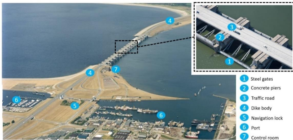
Figure 10 Overview of the components of the Haringvliet sluices. Photo edited from (Land+Water, 2020)
