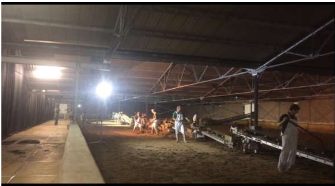
Figure 3: Cleaning of a full scale filter at Scheveningen, Dunea NV
