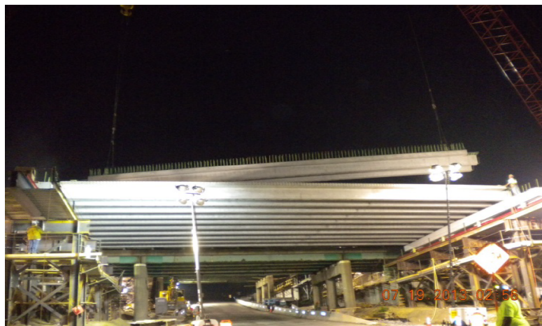
FIGURE 4.8: Erection of the prefabricated superstructure elements [Federal Highway Administration, 2014a]
