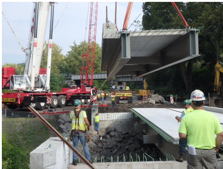
FIGURE 6.2: Prefabricated modular superstructure element placing [Roads and Bridges, nd]
