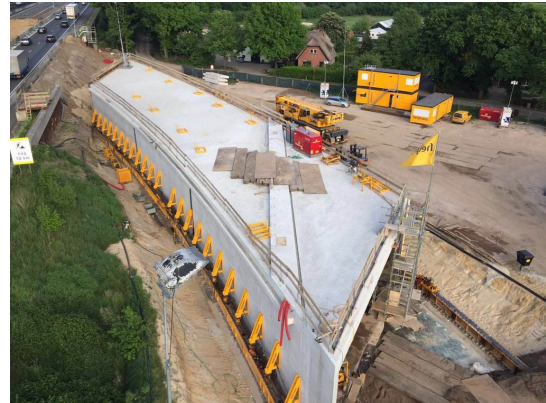
FIGURE 4.27: Lateral slide-in tunnel part in A12 Ede before movement [Heijmans, 2016]
