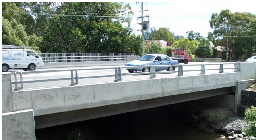
FIGURE 4.34: Shepherd's Gully Bridge, Australia [VSL, 2008]
