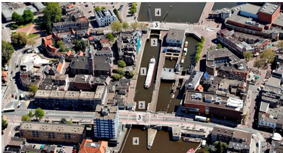
FIGURE 4.48: Overview of the Wilhelmina lock, with at the top (south) the Beatrix Bridge and at the bottom (north) the Wilhelmina Bridge [van Cann et al., 2017]
