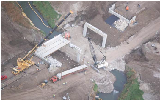
FIGURE 4.5: Prefabricated steel/concrete module [Federal Highway Administration, 2013]
