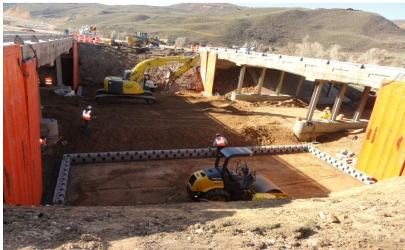
FIGURE 4.18: Construction of the median substructure with GRS-IBS [Federal Highway Administration, 2014b]
