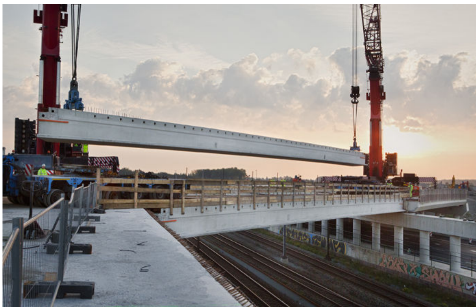
FIGURE 4.25: Erection of prefabricated bridge girders in A9 Badhoevedorp [Spanbeton, nd]
