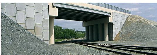
FIGURE 4.38: Saint Pierre La Cour Bridge, France [Ductal, nd]
