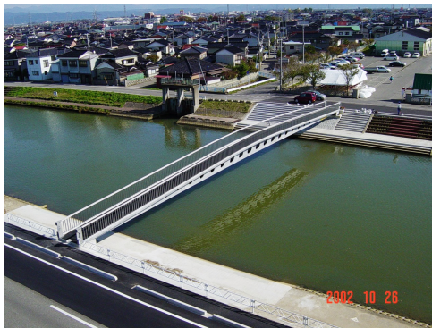
FIGURE 4.32: Sakata-Mirai Footbridge, Seoul, South Korea [VSL, ndb]
