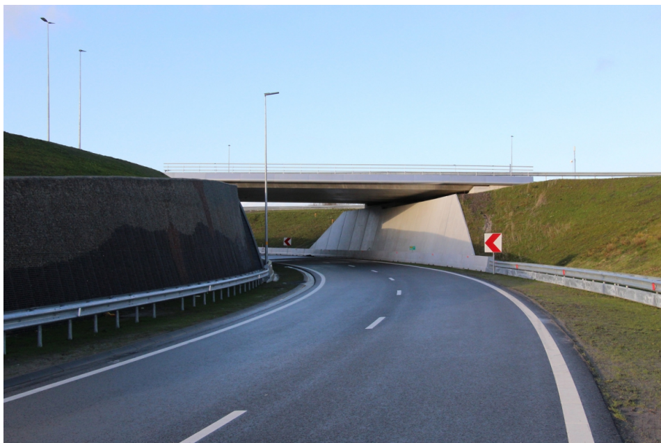
FIGURE 4.24: Retaining structure in reinforced soil [Geolics, 2015]
