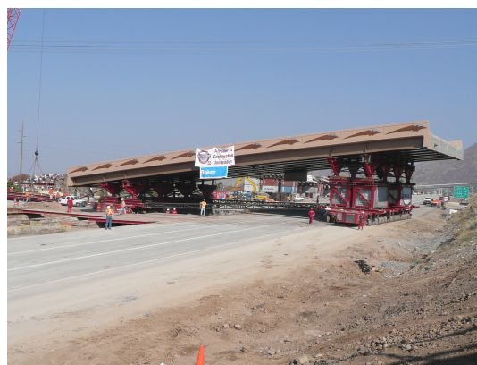
FIGURE 6.4: Superstructure placement by means of a SPMT [Florida International University, ndd]
