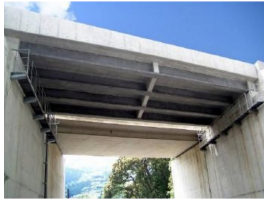
FIGURE 4.40: Horikoshi C-ramp Bridge, Japan [Resplendino and Toulemonde, 2013]
