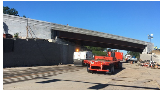
FIGURE 4.23: Final situation after the bridge replacement [WPRI, 2016a]
