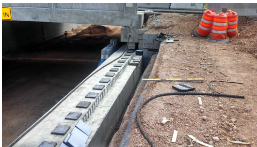
FIGURE 4.20: Lateral slide-in layout for the eastbound bridge [Federal Highway Administration, 2014b]
