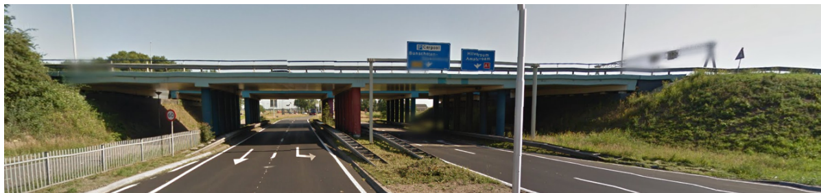
FIGURE 10.1: Google street view of viaduct Zeldert
