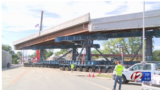
FIGURE 4.22: Superstructure movement by SPMT to the bridge location [WPRI, 2016b]
