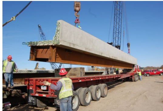
FIGURE 4.4: Erection of the prefabricated modules [Federal Highway Administration, 2013]
