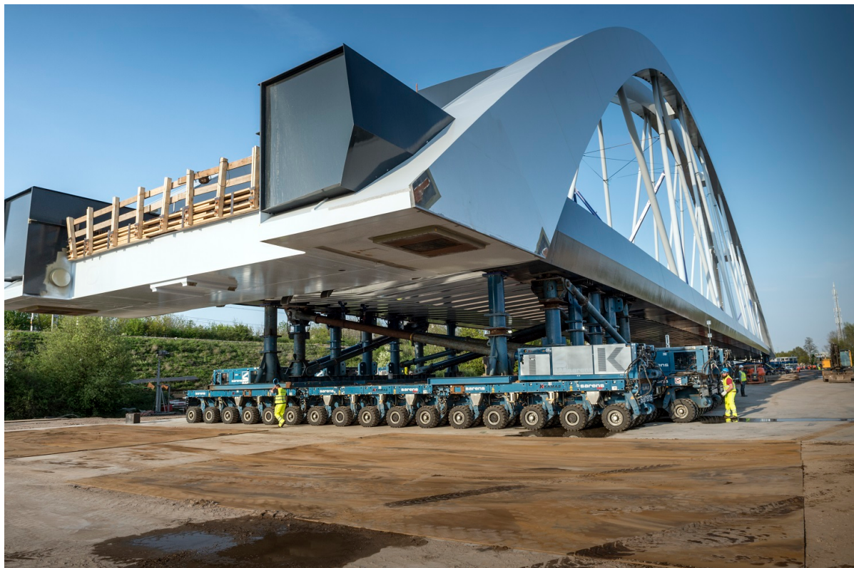
FIGURE 4.28: Railway bridge Muiderberg during movement by SPMT's [Rijkswaterstaat, ndc]
