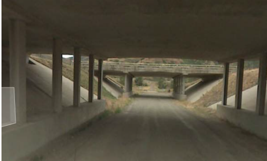
FIGURE 4.16: Underpass situation prior to bridge replacement [Federal Highway Administration, 2014b]
