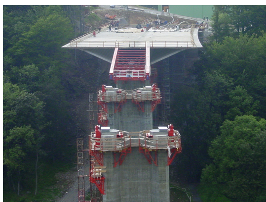
FIGURE 6.5: Incremental bridge launching technique [VSL, nda]
