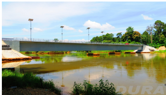
FIGURE 4.43: Batu 6 Bridge, Malaysia [DURA, 2015]
