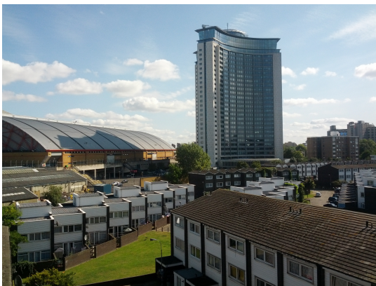
FIGURE 4.45: The Empress State Building [Wikipedia Commons, 2012]
