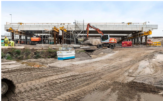
FIGURE 4.26: Lateral slide-in railway deck in A9 Gaasperdammerweg before movement [Rijkswaterstaat, ndb]
