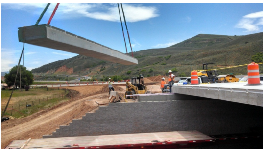
FIGURE 4.19: Erection of the superstructure from prefabricated elements [Federal Highway Administration, 2014b]
