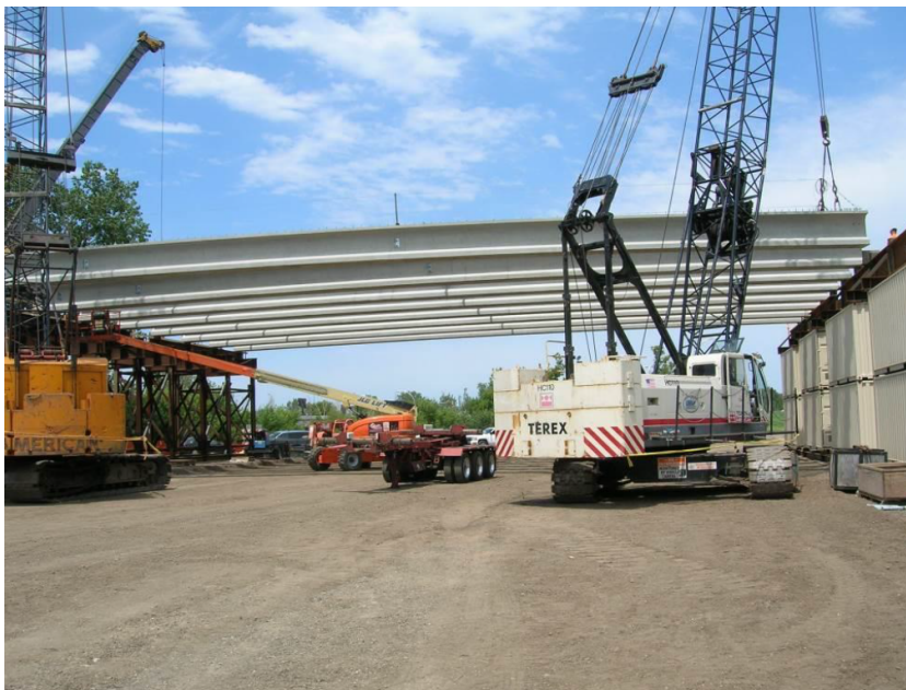
FIGURE 4.12: Off-site erection of the prefabricated superstructure [Federal Highway Administration, 2015b]
