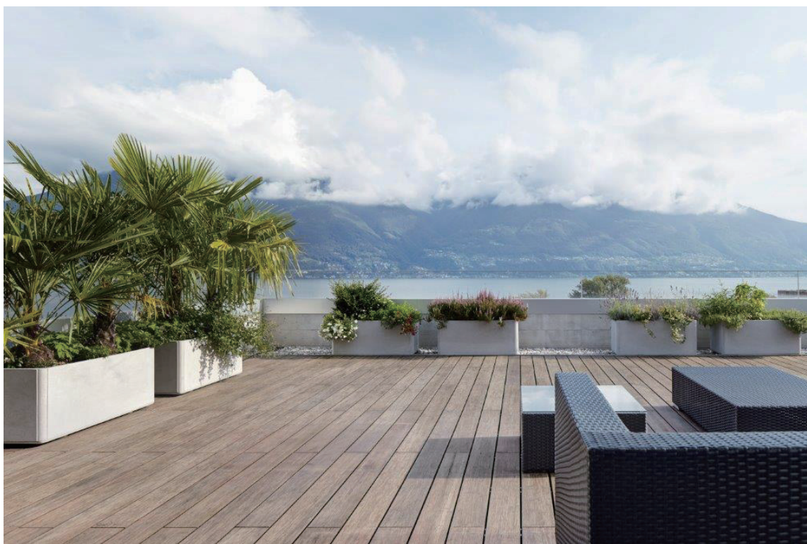
Figure 3: Thermally modified exterior SWB decking, Switzerland. (Photo credit: Danielle Kahr / MOSO International)
