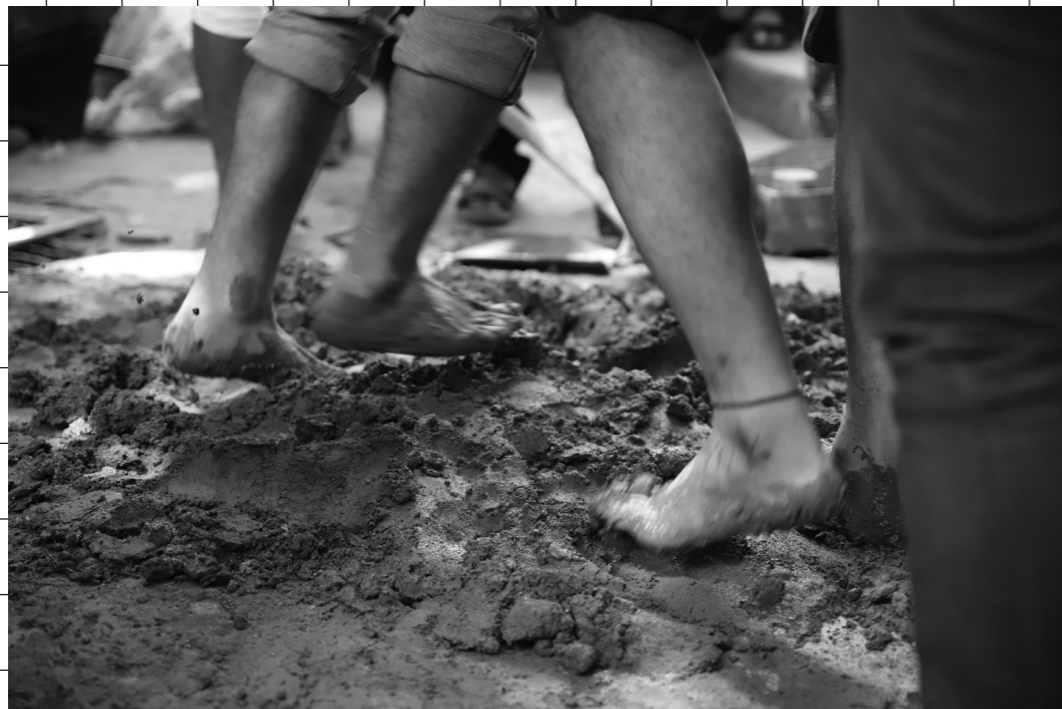
Students pugging mud at the 'Building with Stabilised Mud' workshop, July 2019, Mjinmayee office, Bangalore. Photograph by the Curt Gambetta.
