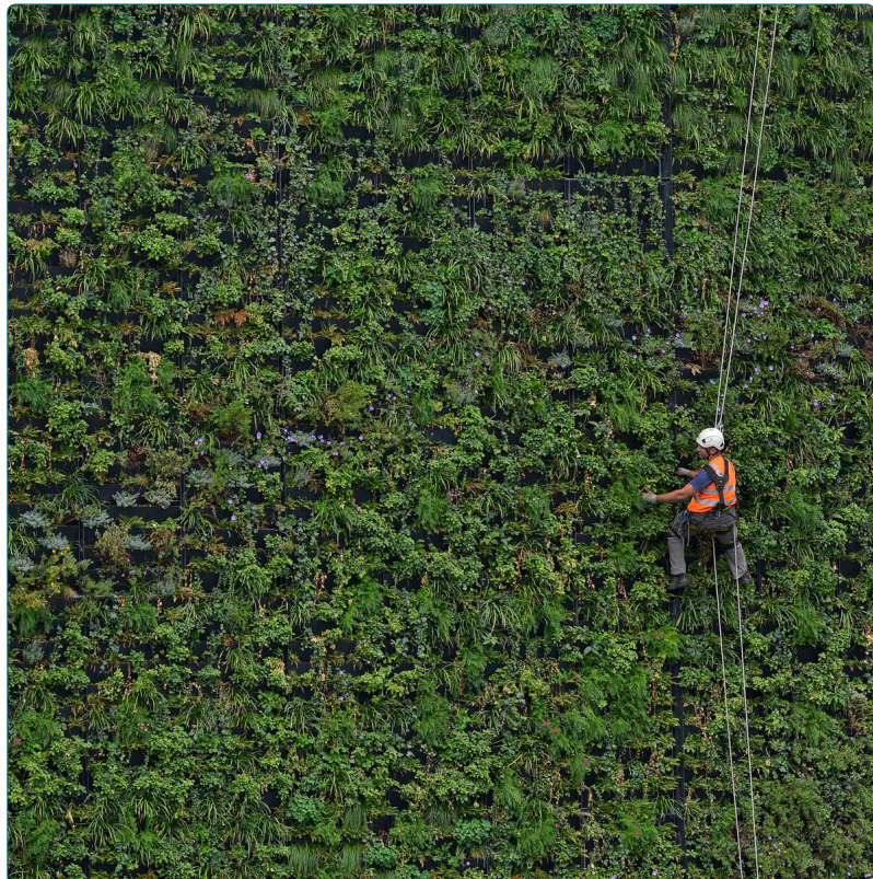
Figure 41 LWS facade maintenance
