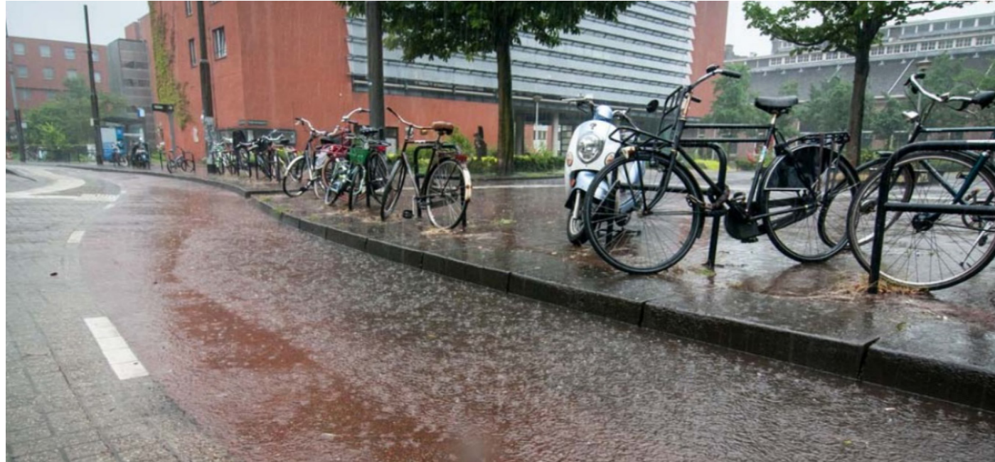
Figure 58 Sidewalk protect against storm water
