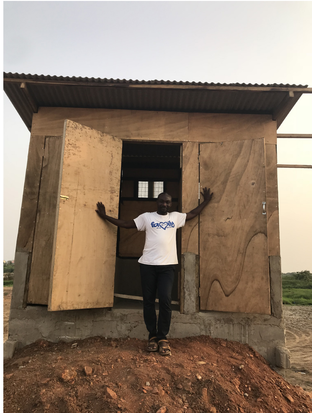
Mr. Philip Seshie shows the new community toilet block.
