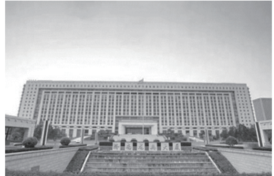
Jinan Municipal Party Committee and Government Office Building. Source: Government Office Buildings in Shandong, Shanghai and Guangzhou.
