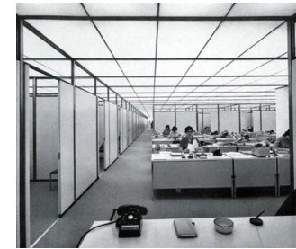
Skidmore Owings and Merrill, Union Carbide Building
